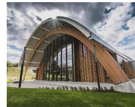
Slough Ice Arena
