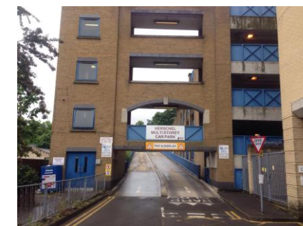
Herschel multi-storey car park
